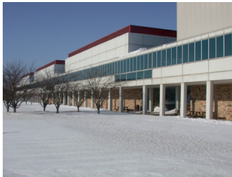
Knoll's Lubin Manuf. Facility, East Greenville, PA Original Architect: Mitchell/Giurgola Architects LEED Consultant: Envision LEED Existing Buildings Pilot Project - Gold Certified
