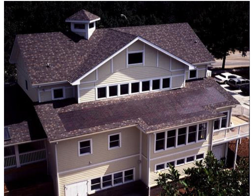
South Face Institute Eco-Green building in Atlanta, with building integrated Photovoltaic roof shingles.
